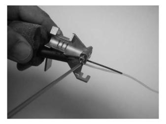
3.6 Remove the redundant strength member as shown.
