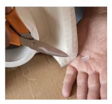
**6.** By removing one or more "teeth", the flexible edge strip can bend to 90°.
