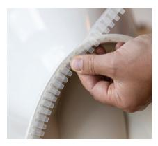
**2.** Place the flexible edge strip onto the toilet, as displayed in the picture, with the sticky side facing down towards the toilet along its outer edge.
