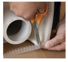
**3.** Cut or shear off any excess edge strip with sharp scissors or a knife so that the edges match.
