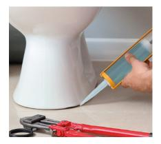
**7.** Once the toilet is fitted, grout it with sanitary silicone.
