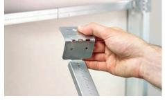
Bend the bracket ends to fix onto the studs.
