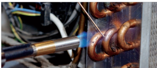
Brazing in aircon and refrigeration
