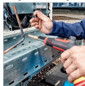
Brazing in aircon and refrigeration
