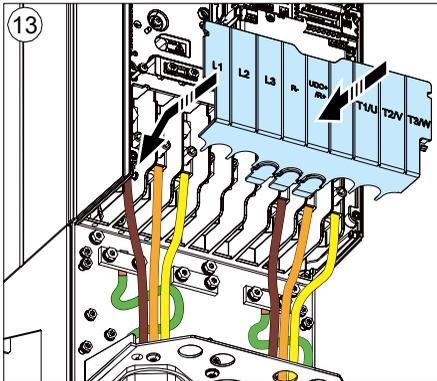
14. Secure the conduits outside the unit mechanically.
